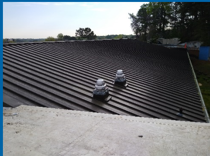
New Standing Seam Metal Roofing Installation
