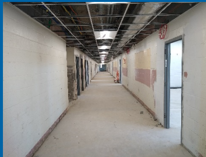
Hang Ceiling Grid and Lights at Building 2010A Corridor
