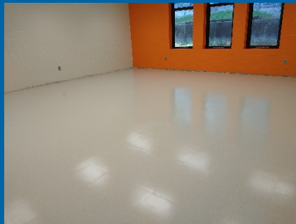
Lay VCT at Building 2021 & Building 2020
